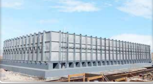
Project Location : Qatar
