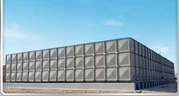
Project Location : Qatar
